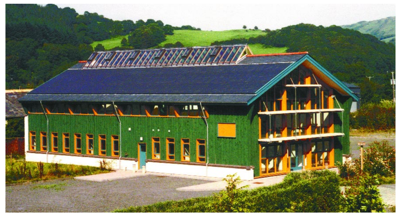
Energy and cost savings were achieved using Onduline roofing sheets for this award-winning building at the Dvfl Eco Park in North Wales
